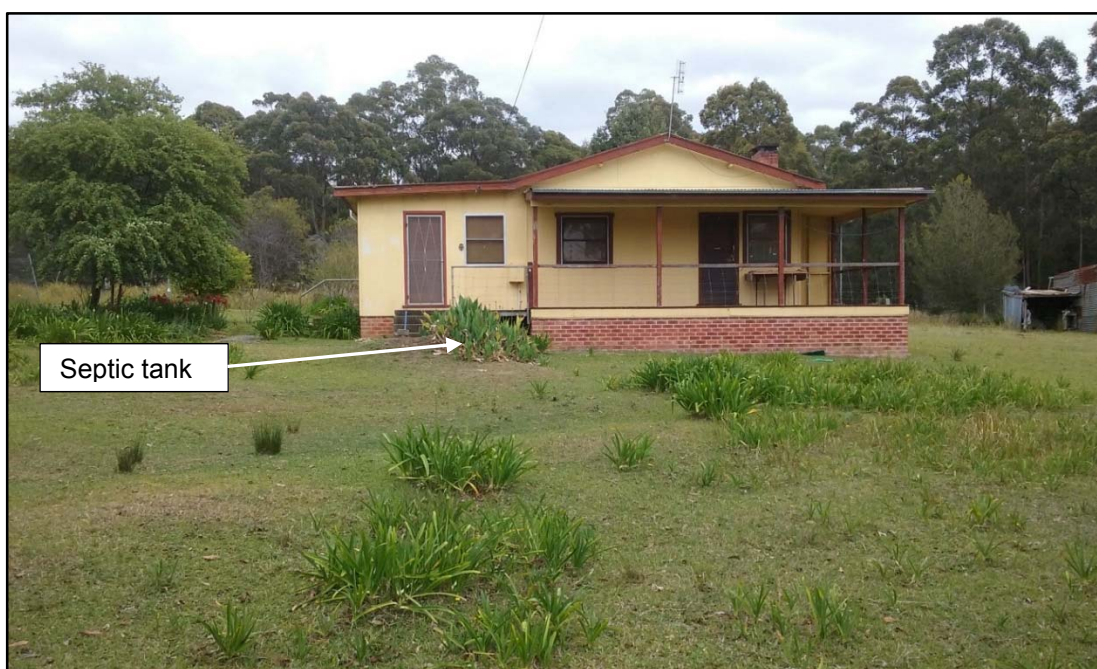
Plate 1: Existing dwelling house and septic tank.
